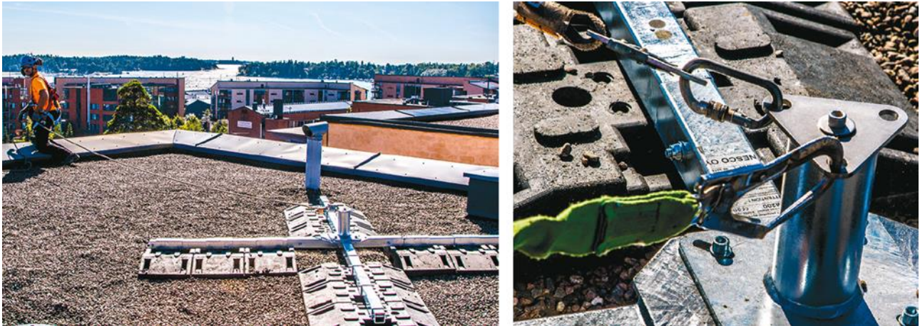
Figure 1. Counterweight anchor, weight 374 kg
