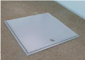
Figure 1. Hatch on the balcony floor
