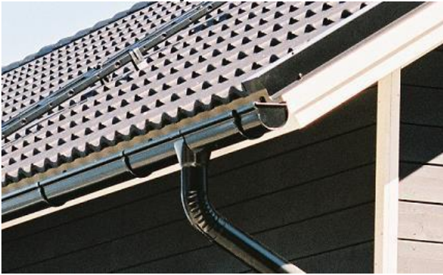
Figure 1. P13 gutter with external fixture and running outlet
