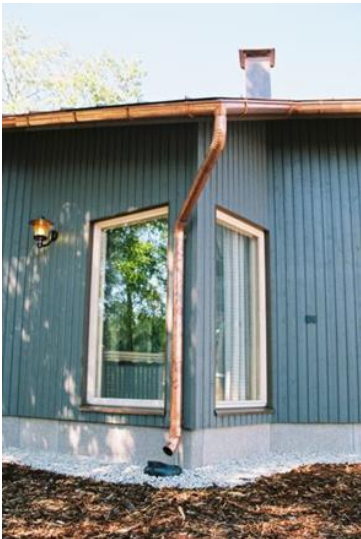
Figure 1. P13 gutter with external fixture and running outlet
