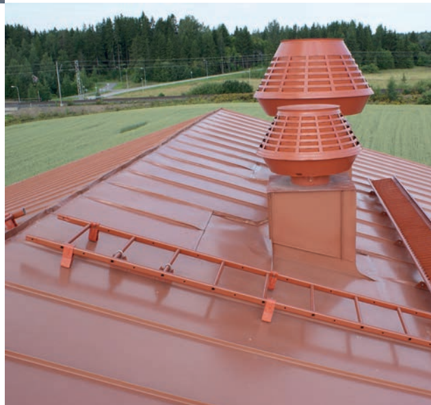
Roof ladders are installed on the roof to secure passage in line with the roof plane.
