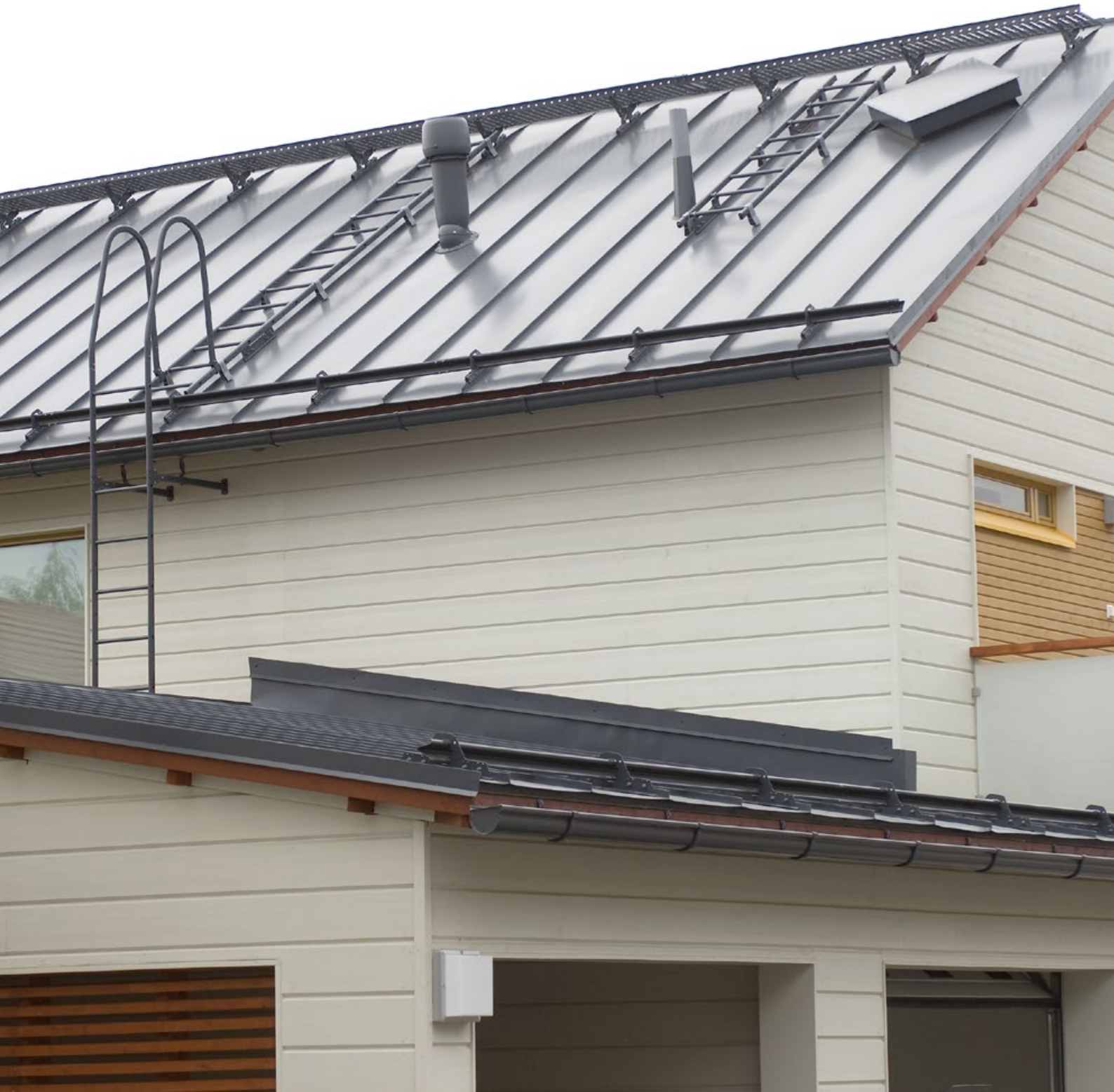
Horizontal rail on a roof walkway
